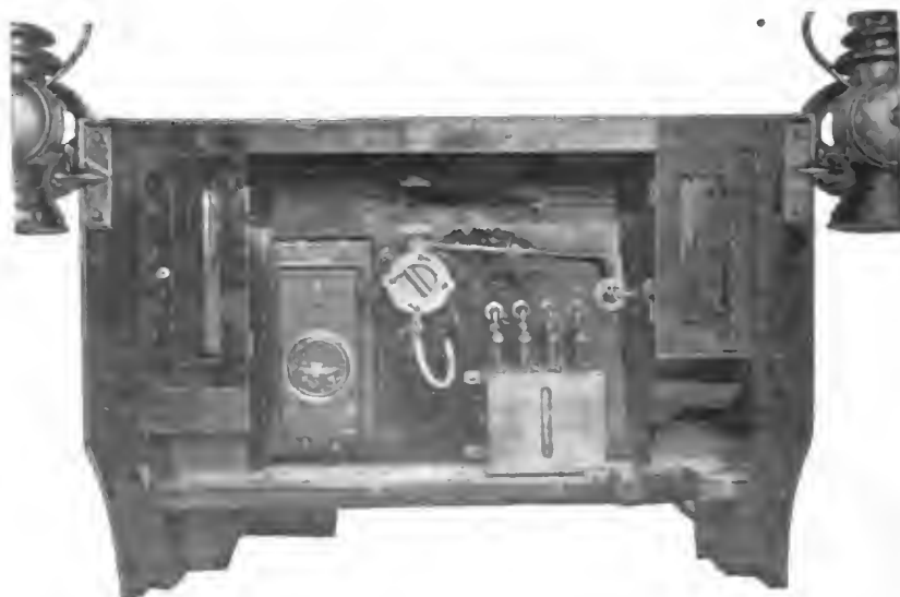
STEEL DASHBOARD OF THOMAS CAR.—TOOL LOCKERS IN UPPER CORNERS. ] ]
